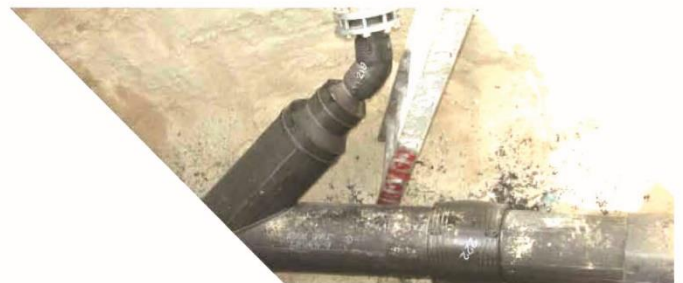
Typical Slip Lining Installation
