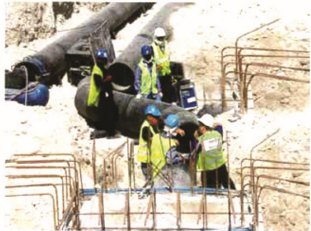
Figure 6-Jointed PE pipes prior to laying
