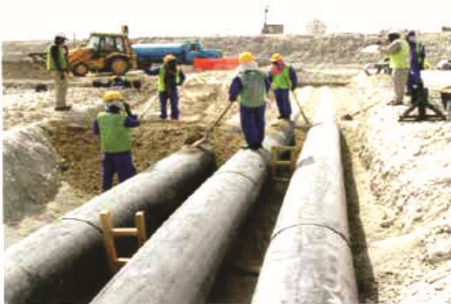
Figure 2-Typical Open Trench
