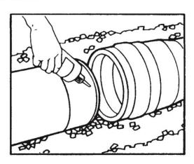
Immediately after lubrication, the spigot \_ should be brought into contact with the socket. The spigot pipe and parent joint should be accurately aligned so that axis of pipes are precisely in line. The spigot should be hand fed into the socket until resistence from the inner sealing selection is felt. Correct alignment at this stage is essential to ensure that the rubber sealing ring is not pinched or torn.
