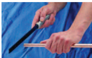
■ Cutting the tube
